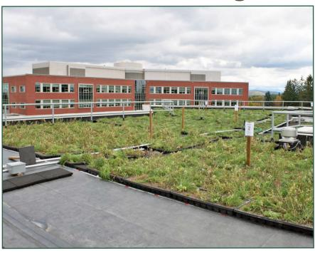
Impervious surfaces, such as pavement and roofs, in urban ecosystems often result in uncontrolled, rapid runoff of stormwater. During runoff events, the high volume of water deposited into waterways carries pollutants from impervious surfaces and silt from erosion and contributes to elevated water temperatures. Green roofs are a new way to reduce stormwater impacts.
