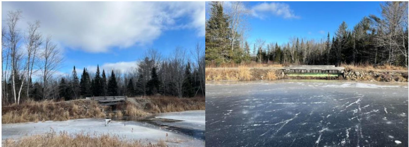
Figure 52. Bridge sites targeted for reconstruction, corresponding to the southern site (left) and the northern site (right). Photos: Kyle Hubbard
