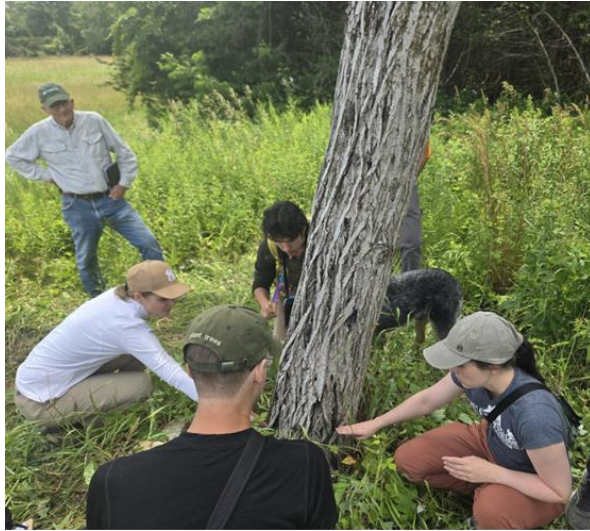
Figure 47. Project participants inspect a butternut tree for signs of the butternut canker disease.
