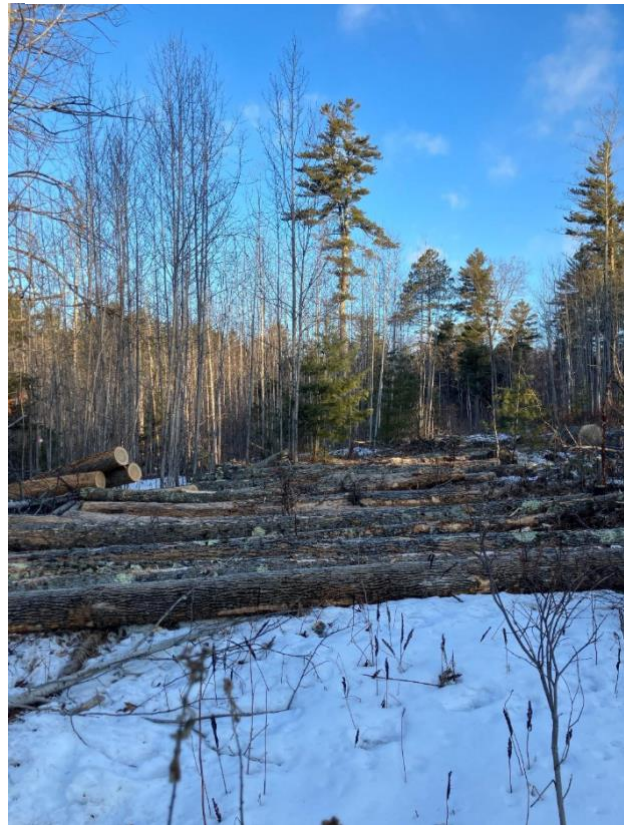
Figure 23. Corduroy installation at Marlboro VT site (photo by Shannon Van Hise)
